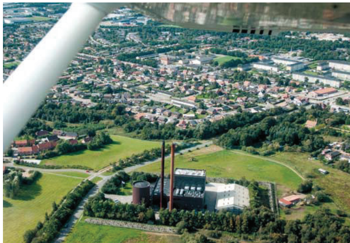
Aerial view of Thorsvej district heating plant (I/S Skive Fjernvarme) in Denmark. ▼
