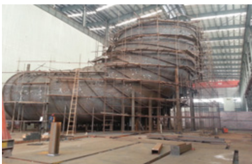
Draft tube installation
