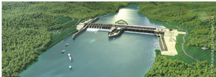
Navigation lock, spillway, intermediate block, powerhouse and fish ladder
