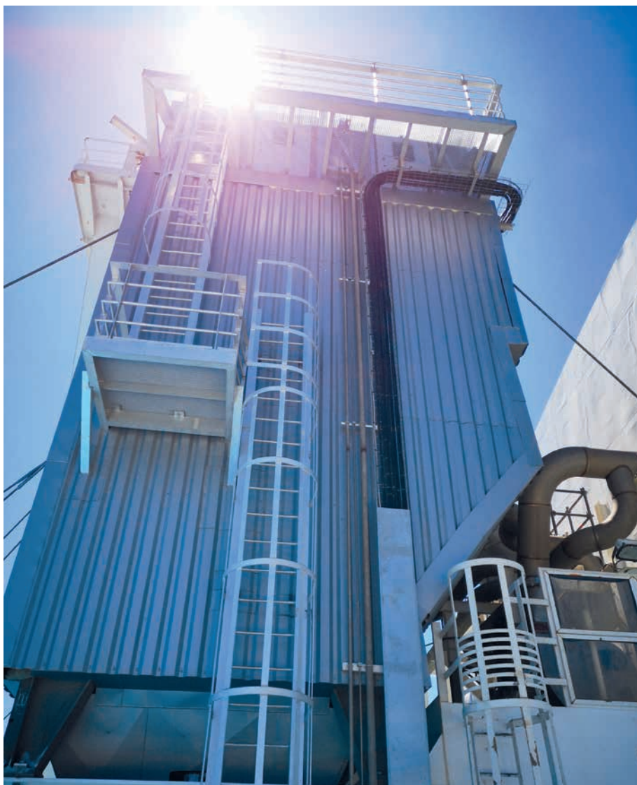
The Andritz SeaSOx dry system installed
