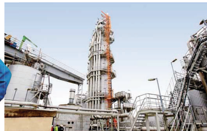
▲ ZPR now gets about 100 t/d more production out of its digester as a result of several small improvement projects. The most recent upgrade to the fiberline was the replacement of the lower extraction screens with new ANDRITZ SureFlow diagonal screens.
