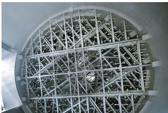
Inner view of an ANDRITZ wet flue gas desulphurization (FGD) scrubber
