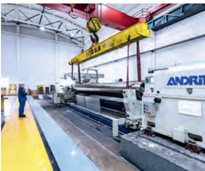
Roll service at the Wuxi facilities
