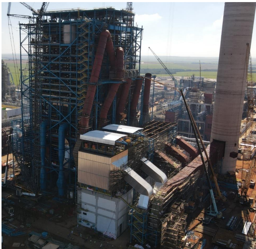
ANDRITZ Recovery Boiler and 5 chamber-ESP under construction
