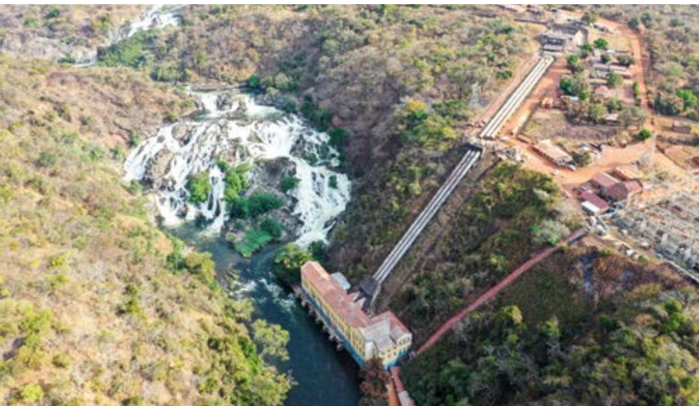
The rehabilitation and modernization will see each unit at Mwadingusha increase output from 11.8 MW to 13.05 MW. The energy will benefit the people of the DRC as well as the Kamo-a-Kakula copper mine.
