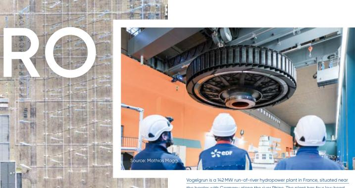
Vogelgrun is a 142 MW run-of-river hydropower plant in France, situated near the border with Germany along the river Rhine. The plant has four low head Kaplan turbines, in service since 1959. During XFLEX HYDRO, one of the units was hybridized with a battery and the performance is being evaluated.
