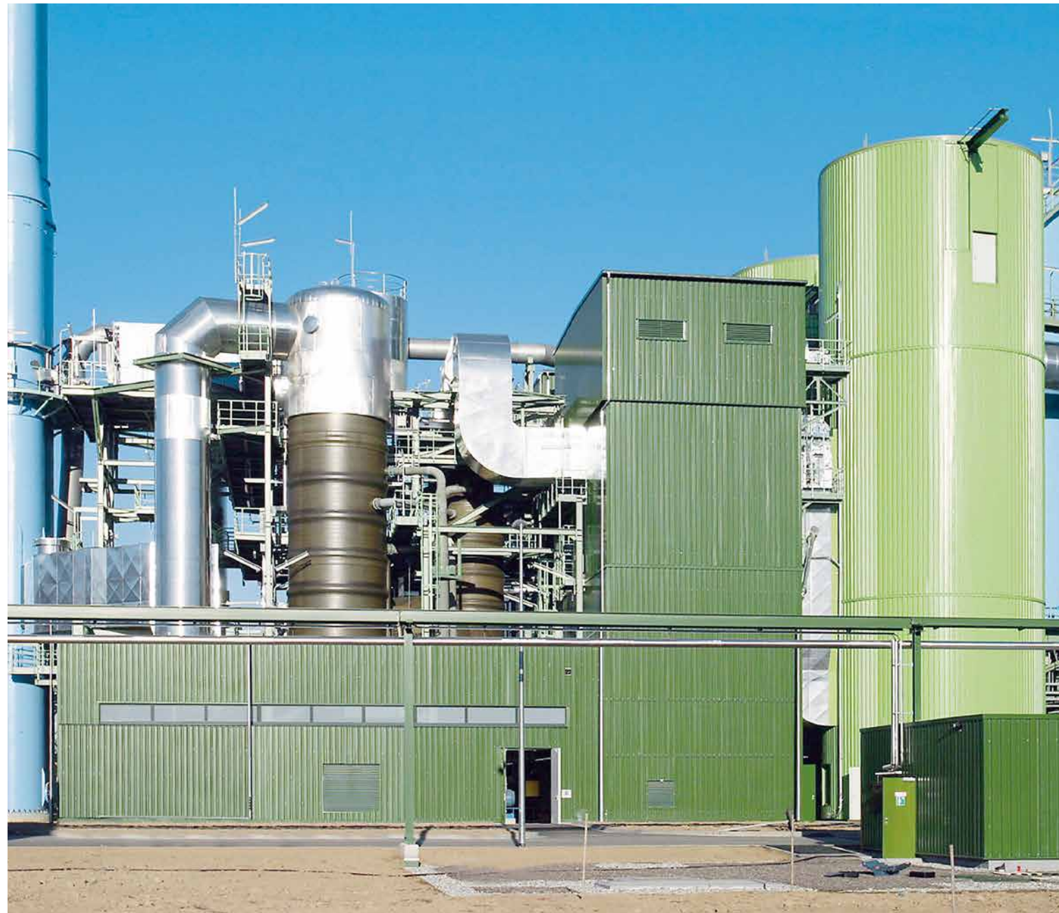
▲ SCR, spray dryer, fabric filter, two-stage wet scrubber, two trains, Mainz, Germany
