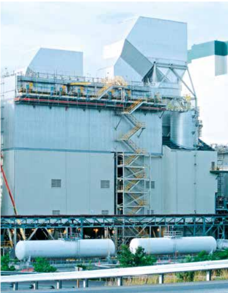
▲ Circulating dry scrubbers (Dry FGD), Virginia, USA
