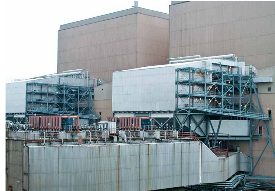
▲ High-dust configuration at Hoosier Energy Merom Power Station, Units 1 & 2, Sullivan (IN), USA
