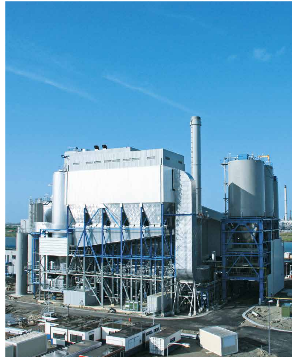
◀ TurboSorp, Fabric Filter, SCR, Moerdijk, Netherlands
