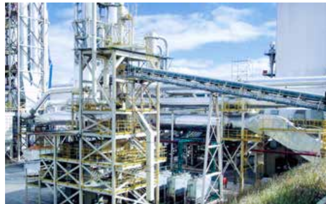
Installation of an ANDRITZ chip washing system
