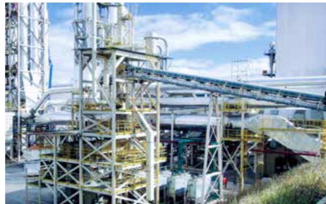
Installation of an ANDRITZ chip washing system
