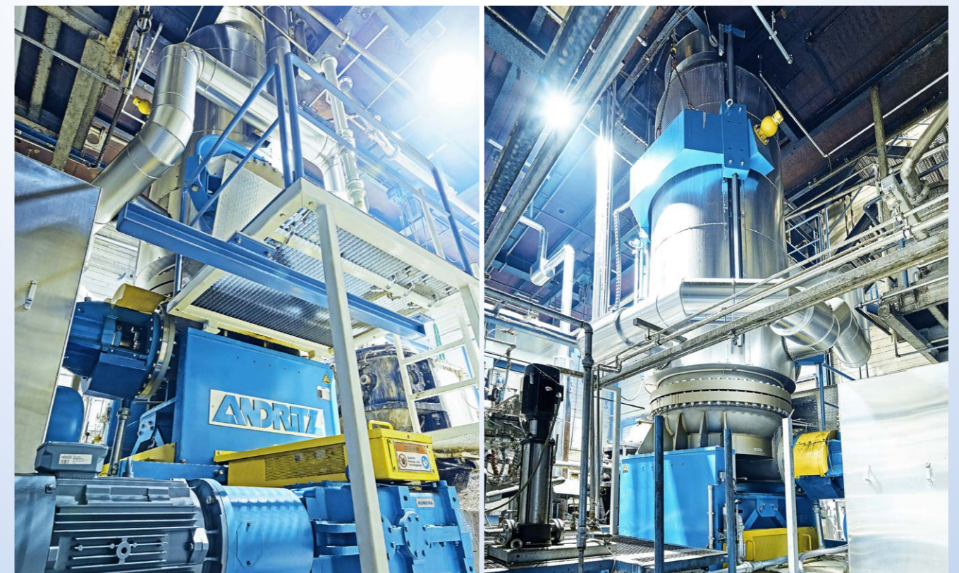
ANDRITZ discharge bottom and digester on-site installation
