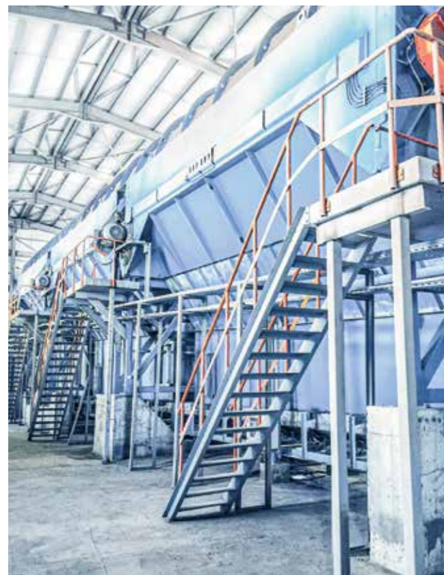
The debarking unit runs around the clock. ANDRITZ trained all operators to run the equipment, which requires only scheduled maintenance at pre-determined intervals.
