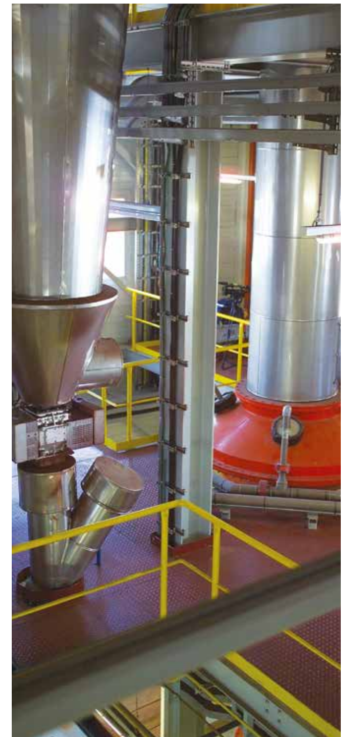
Dust separator and injection of waste pickle at the evaporator
