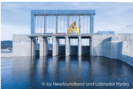
Intake gates including trash racks
