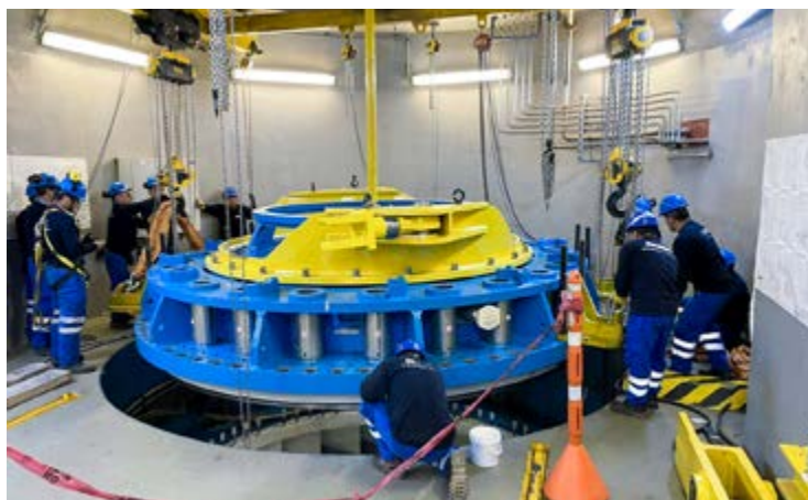
Installation of guide vane apparatus at Cerro del Águila hydropower plant
