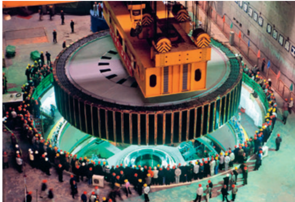
Generator for San Xia, China.
