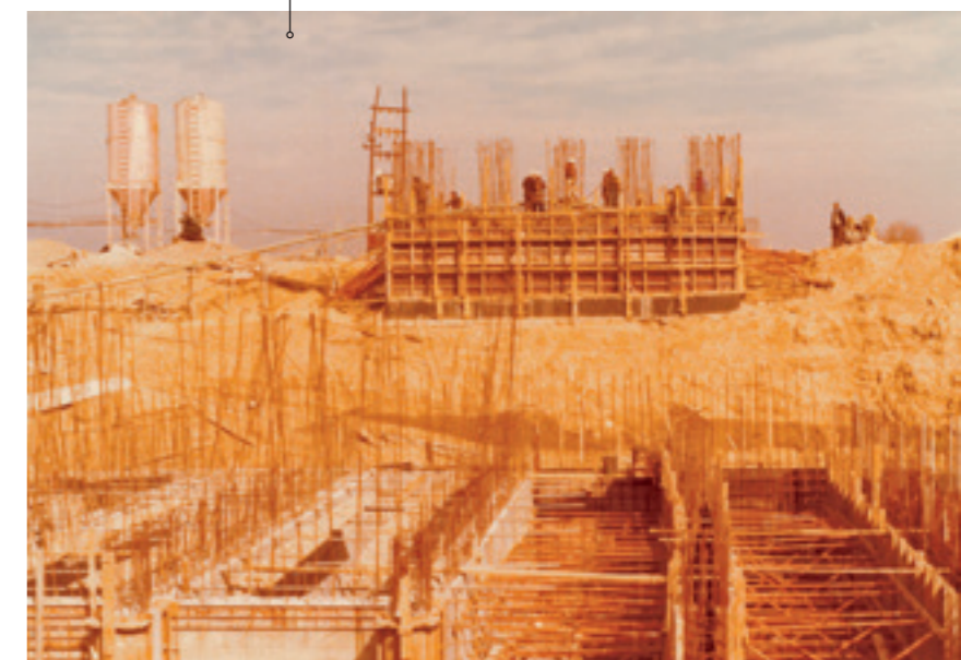
Pump construction in Iraq, 1979.
