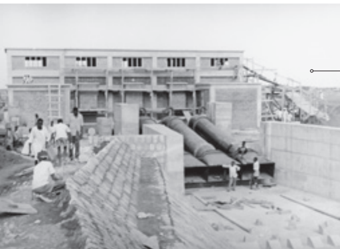
Installation of pipe system in Sudan, 1967.
