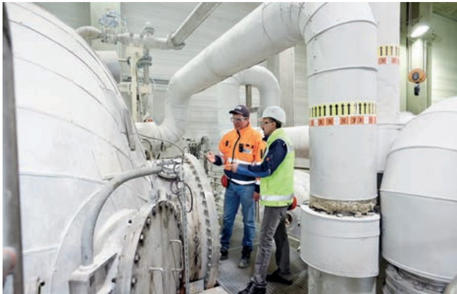
▲ Patrick Ludwig, Production Engineer for Zellstoff Stendal (left), discusses improved performance of the ANDRITZ CD Filter (white liquor filter) after the upgrade with Walter Scholz-Sommerbauer, ANDRITZ Key Account Manager.
