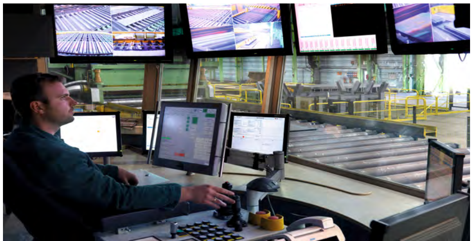
▲ Main operator room
