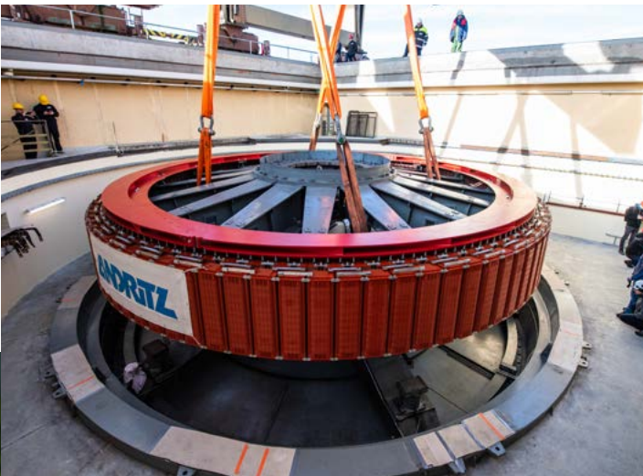
Lowering of generator rotor at the Wallsee-Mitterkirchen power plant. @Johannes Wiedl
