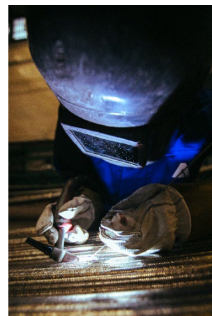
Overlay welding on membrane wall
