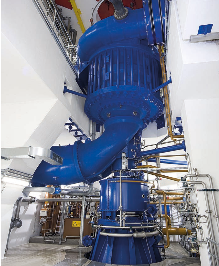
Pump turbine unit with four stages
