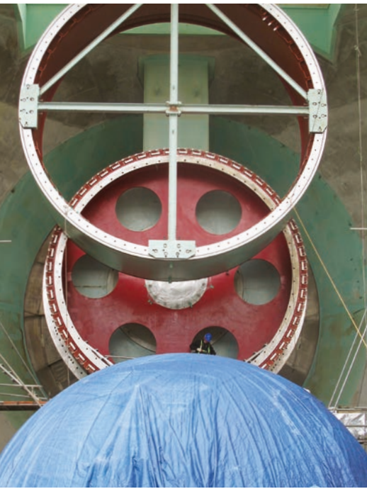
Installation of Bulb Turbine parts at HPP Sihwa, South Korea
