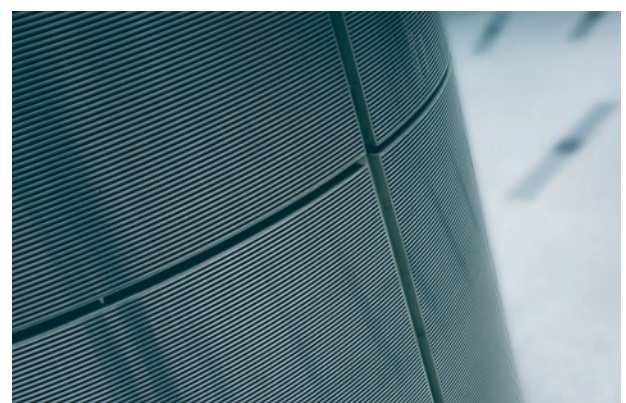
Column panels assembly
