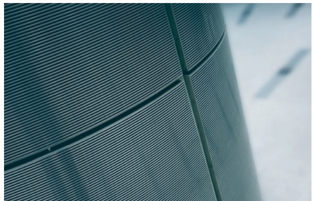
Column panels assembly
