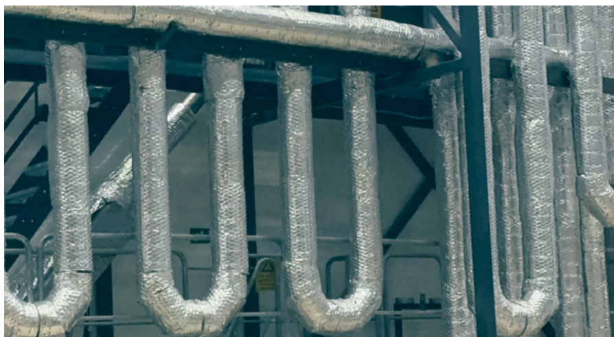
The flash drying pilot facility in Växjö expands ANDRITZ's capabilities in advanced drying technologies for fibers and particulate materials.
