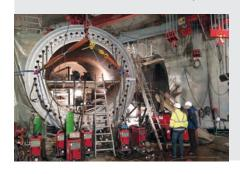
The main installation works at the penstocks, including the filling test, were finished on time in May 2015. In total, about 9,100 tons of steel of different grades and thicknesses have been used and welded during this project. Connection work from the old to the new pressure shaft was carried out between March and April 2016, when the seal on the disc valve was also replaced.
