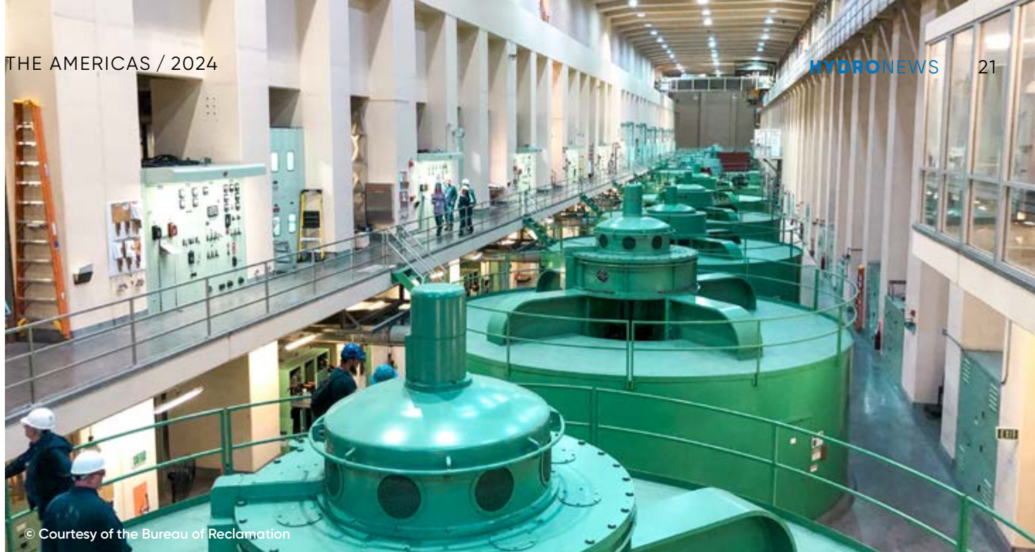
Unit hall of John W. Keys III pumped storage plant at Grand Coulee hydropower complex
