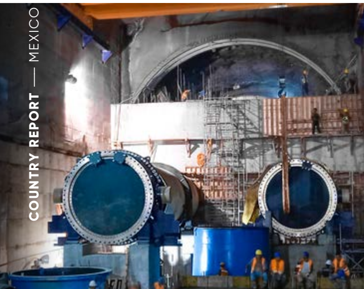
Butterfly valve installation at Santa María hydropower plant
