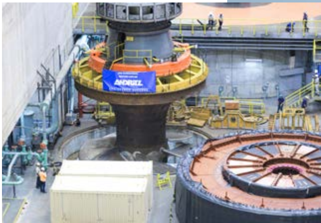
Outside view (right) and installation work of Kaplan turbine (above) at Sobradinho hydropower plant on the São Francisco River, Brazil
