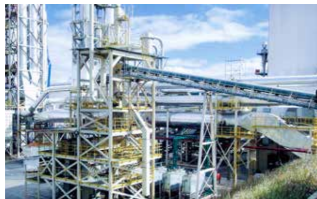
Installation of an ANDRITZ chip washing system
