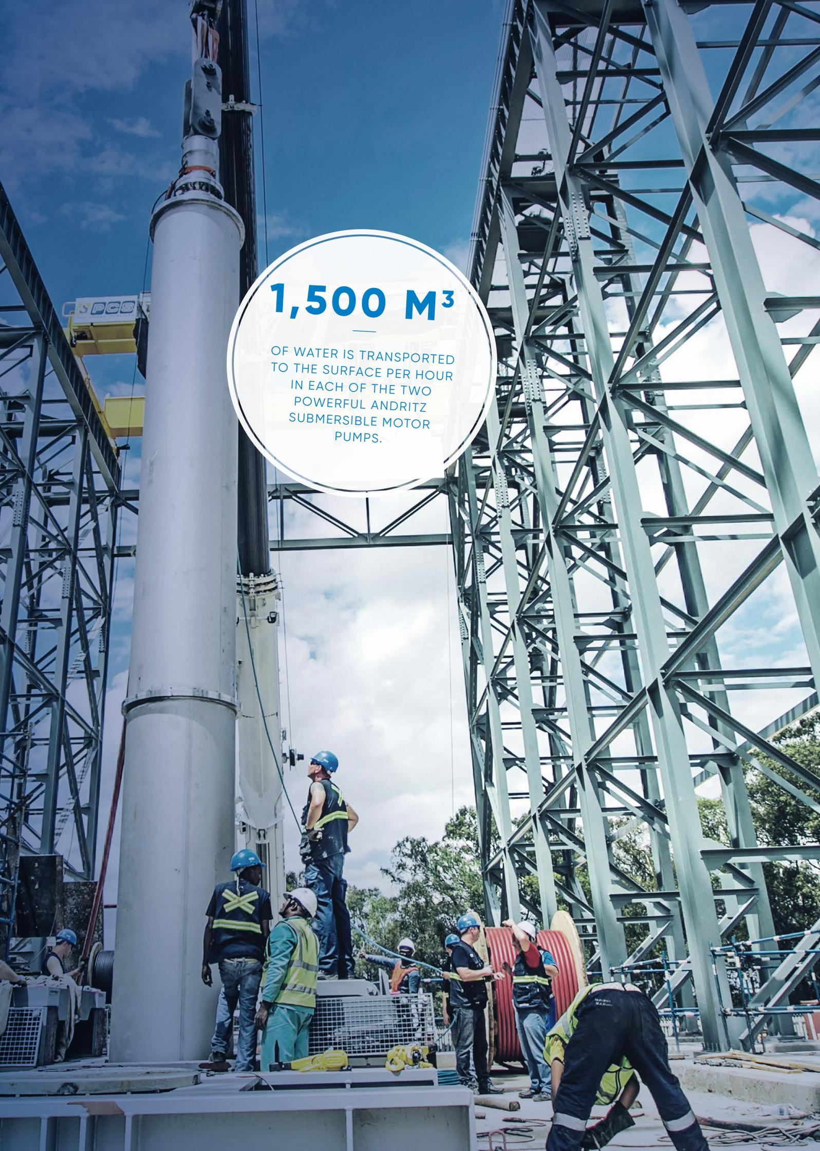
A large white cylindrical pump is being lowered into a complex steel lattice structure. Several workers in safety gear are visible around the base of the structure. The scene is set outdoors under a blue sky with some clouds. A yellow crane arm is visible on the left side of the frame.
