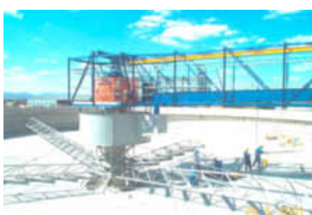
40mØ half span bridge
