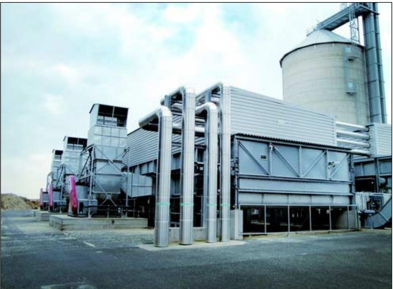
The supplied belt dryer for drying sawdust consists of two BDS-110-S-8.0 (belt drying) lines, each with a water evaporation capacity of approx. 11 tons.
