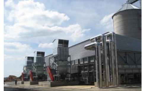
The sawdust to be dried is fed into two symmetrically arranged augers that ensure an even height of the moist material across the whole width of the drying belt. The drying belt moves the material through the dryer where it is heated by means of warm air and dried in the process. At the end of the drying belt, the dry product is moved to the conveying units for further transport by means of a screw discharger.
