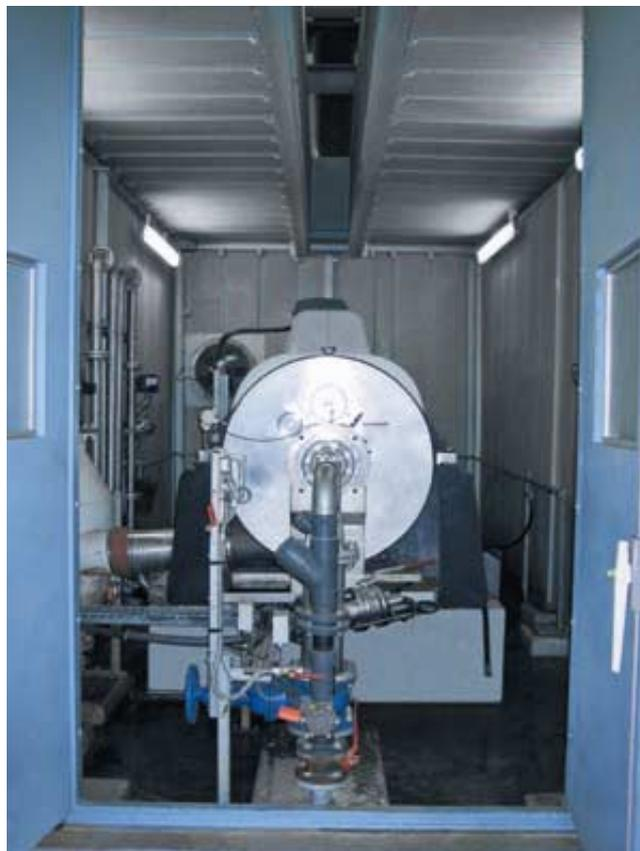
**The Seine Aval wastewater treatment plant in Paris is the largest plant of its kind in Europe and the second largest worldwide, treating the wastewater from six million inhabitants. Four new ANDRITZ decanter centrifuges will help the operator meet reduced nitrogen levels as of 2011.**
